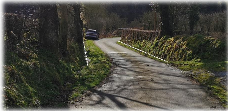
Figure 2.1 – Open Drain Channels
